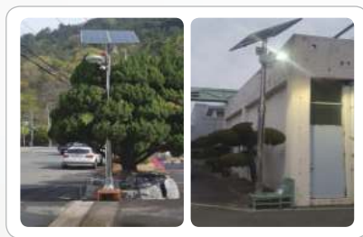
Security Control System
