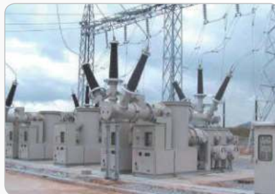
High Voltage Circuit Breaker CB Mechanism and others
